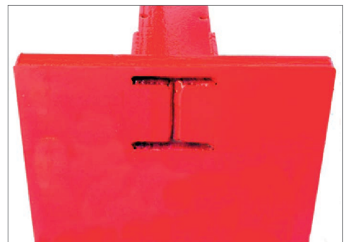
For robustness the steel beam is set into the non-skid plate and welded on both sides
