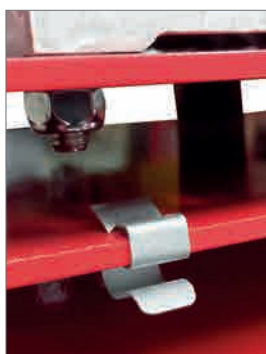
Cable grommet to protect the lighting cable
